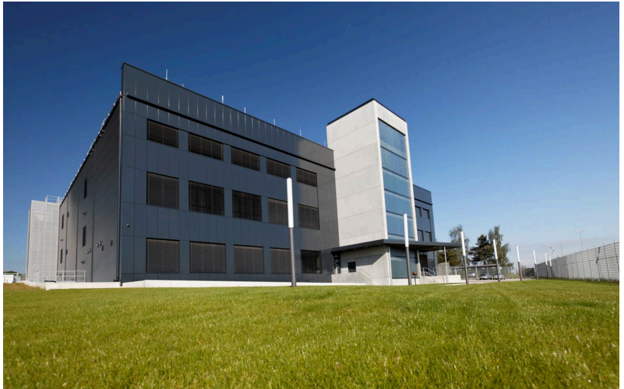
DATA CENTER Netcloud, Rümlang (Foto e-Shelter)
